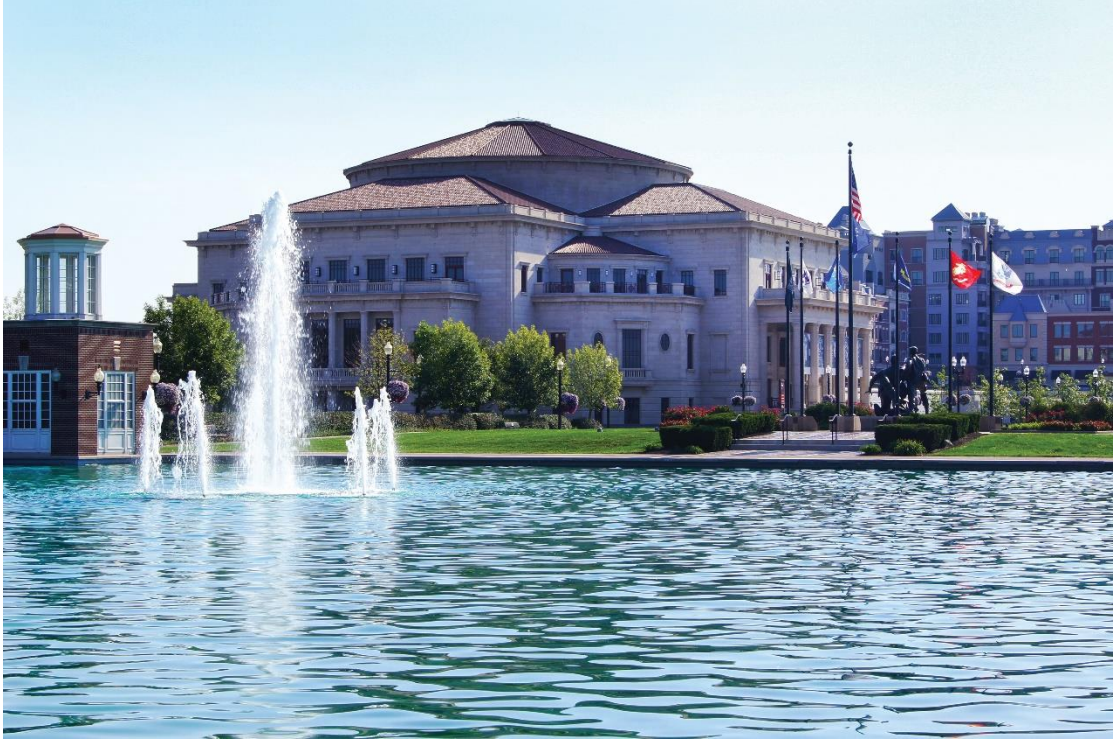
Photos 1. Carmel Performing Arts Center
